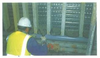
✓ If excess grout builds up on the walling and supports it is good practice to lightly brush these clean before the concrete hardens.
